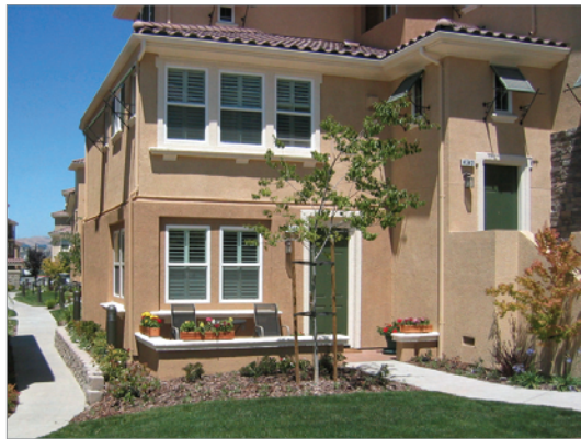
Figure 3.B.38: Units and porches can step down to grade to hide the parking podium behind
