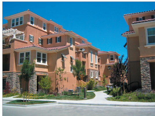
Figure 3.B.45: Good Example of Rooflines - Eaves Create Shadow Line and Form that Relates to Interior Use
