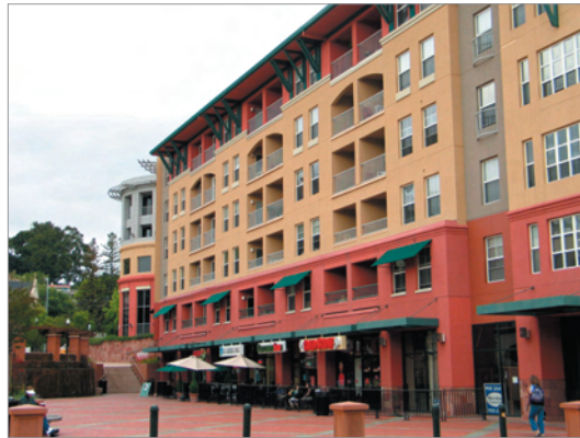
Figure 3.A.4: Buildings should create a direct relationship to sidewalks, plazas, and open spaces to take advantage of the activity in these spaces with ground floor retail or other active uses.
