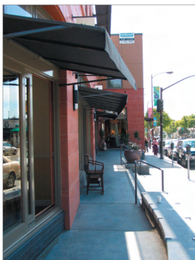
Figure 3.A.42: Canvas awnings along these shop fronts provide a comfortable and shaded space for pedestrians to sit and rest, eat, or watch activity along the sidewalk.
