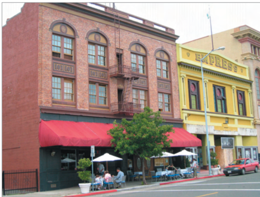
Figure 3.C.59: A Well-Defined Building Wall.
