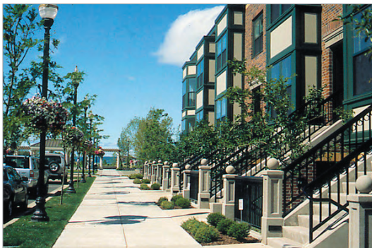
Figure 3.A.8: Multi-family buildings can have individual unit entries accessed directly from the street.
