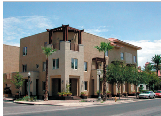
Figure 3.A.24: (Example of Poor Design) Roofs that are devoid of interest create abstract buildings that are less engaging to pedestrians.
