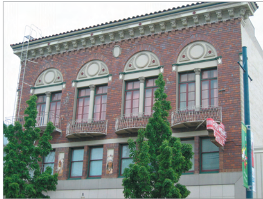
Figure 3.C.80: Juliet balconies can be found on buildings in Vallejo's Downtown.
