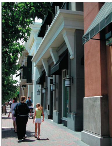
Figure 3.A.27: Exaggerated and over-sized architectural detailing creates caricature buildings.
