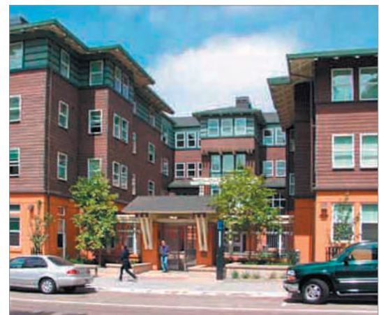
Figure 3.A.19: A well-defined base, middle, and top grounds the building and creates a distinct and identifiable termination with articulated eave.
