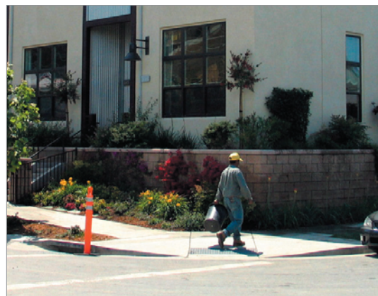
Figure 3.C.69: (Example of Poor Design) Planters should not exceed a comfortable pedestrian-scaled height. These are too tall.
