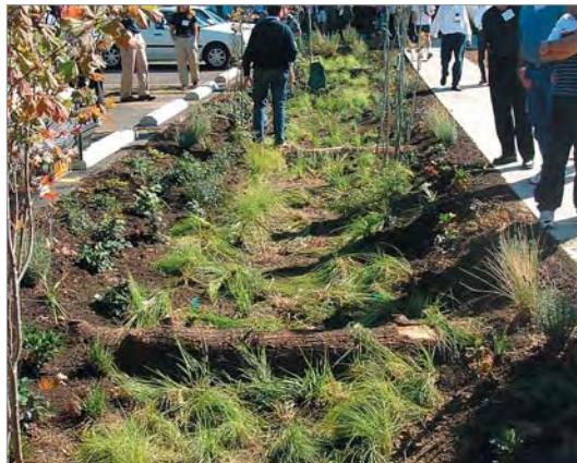
Figure 3.D.65: Example of Swale with Ornamental Planting
