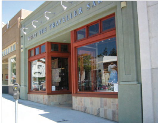
Figure 3.A.37: Retail with High Ceiling and Transom Windows
