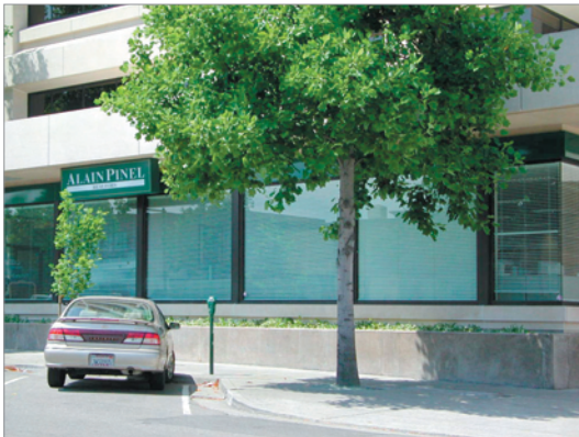
Figure 3.A.33: (Example of Poor Design) Care must be taken to avoid situations where office blinds are frequently drawn to create some privacy.
